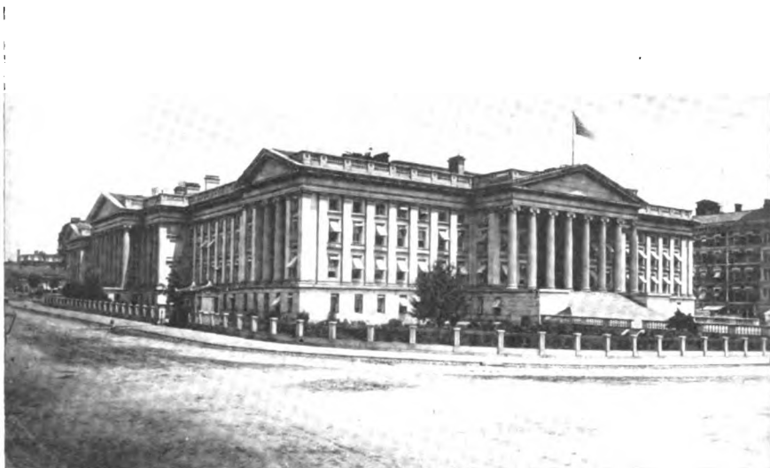
Treasury Building, 1909. South and West Fronts.
